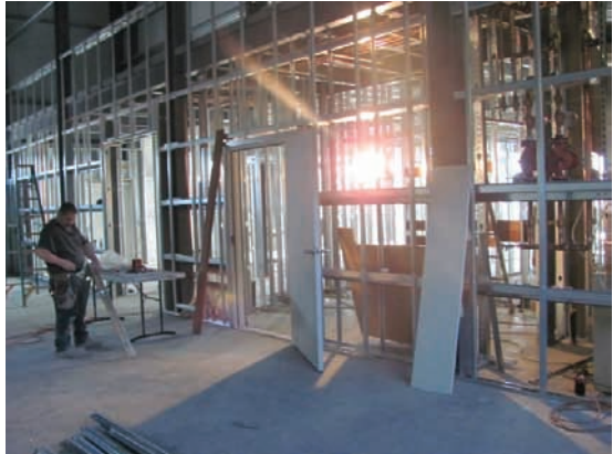
In February the interior framing was completed for the Heritage Center
